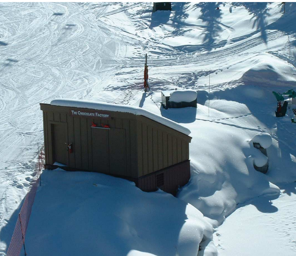
Aerial photograph of the Aspen Ski Company's Powerhouse, Colorado, USA
